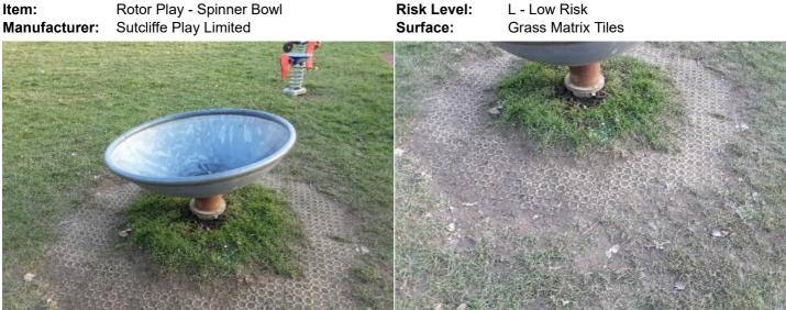
Finding: The grass mats are silted up and the soil is compacted; this may have an effect on the impact absorbing ensure the correct surface qualities are maintained for the properties of the surface
