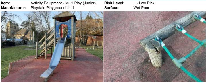
**Finding:** There are splits in the timber running through fixing **Action:** Replace all affected timber parts points and creating some instability in the structure
