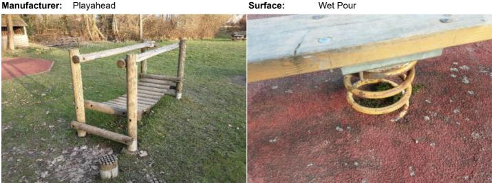
Finding: The paintwork on the spring has been damaged or Action: Treat any rusting components and repaint worn exposing the metal underneath which is rusting
