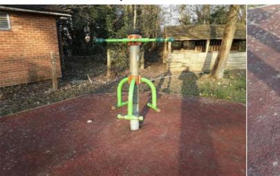
Finding: The paintwork on this item has been damaged or Action: Treat any rusting components and repaint worn exposing the metal underneath which is rusting
