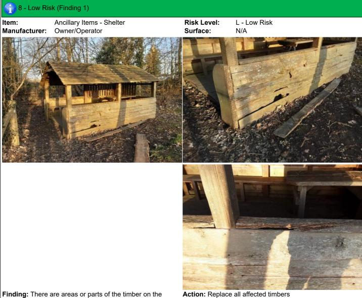
**Finding:** There are areas or parts of the timber on the structure that have rotted
