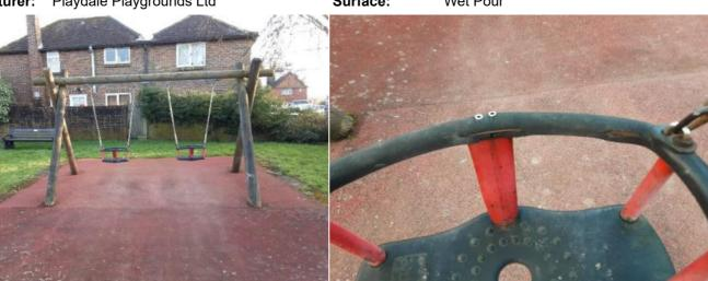
Finding: The swing seat frames are corroding
