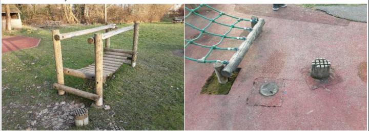
Finding: The adjacent log beam forms a hard object within Action: Monitor - No remedial work recommended the falling space of the equipment in contravention of the requirements of BS EN 1176 Part 1
