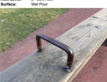
Finding: The paintwork on this item has been damaged or Action: Treat any rusting components and repaint worn exposing the metal underneath which is rusting
