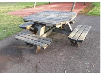
Finding: The table/s is/are not secured to the ground and there is some potential for the item/s to be moved within falling spaces of equipment
