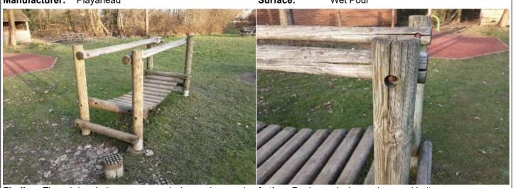
**Finding:** There is/are bolt cap covers missing or damaged on the item
