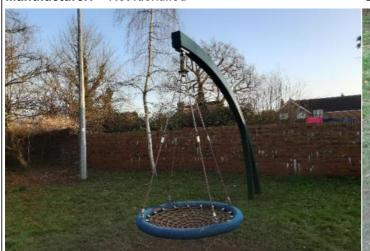
**Finding:** The incorrect seat design has been installed on this swing; there are unique designs for Type 1 and Type 3 swings that provide differing impact attenuating properties to the leading edges of the seat and/or has incorrectly aligned seat eye fixings which will lead to accelerated wear.
