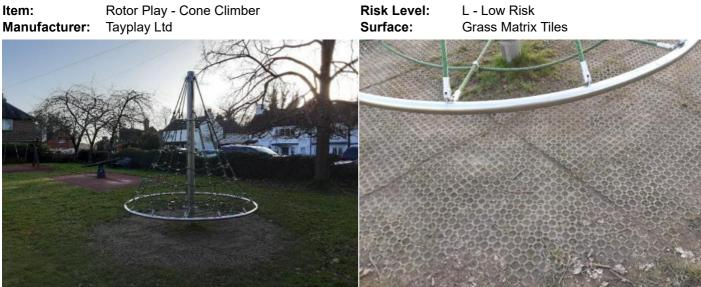
Finding: The grass mats are silted up and the soil is compacted; this may have an effect on the impact absorbing ensure the correct surface qualities are maintained for the properties of the surface
