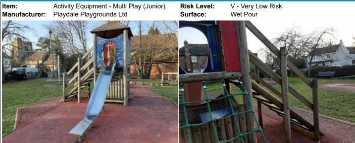
**Finding:** There is insufficient guarding on the steps leading **Action:** Monitor - No remedial work recommended up to the platform that exceeds 1m in height which contravenes the requirements on BS EN 1176 Part 1
